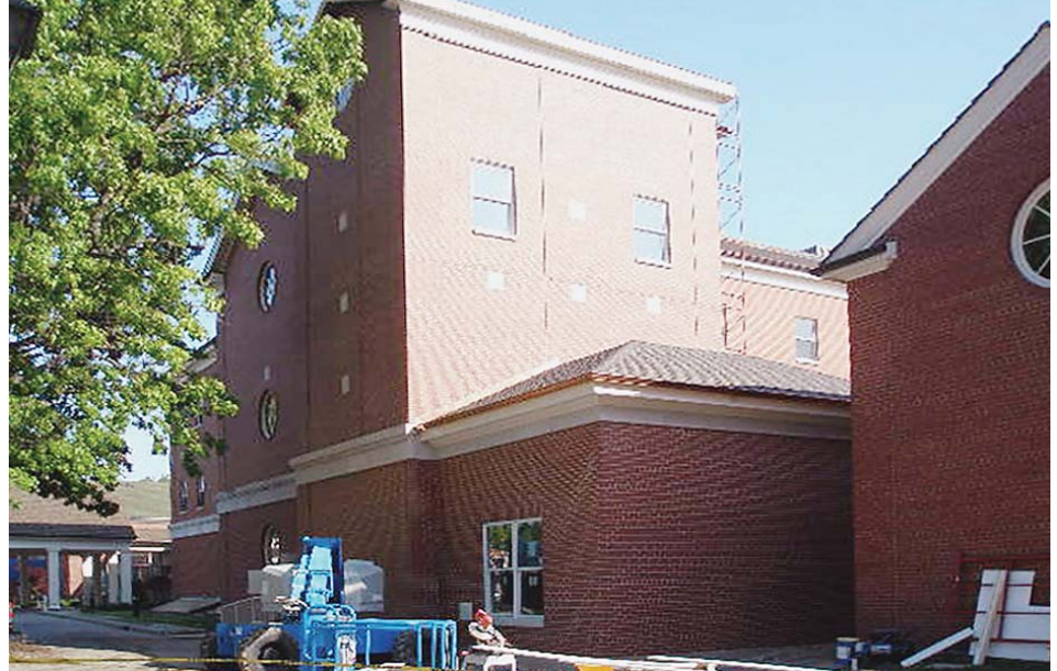
The new addition at Missouri Delta Medical Center.
